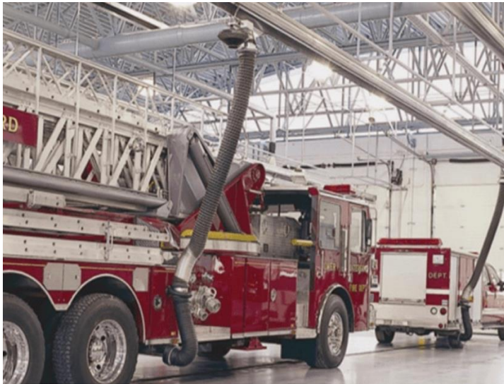
Figure 7. Diesel exhaust extraction device commonly used in fire stations.
