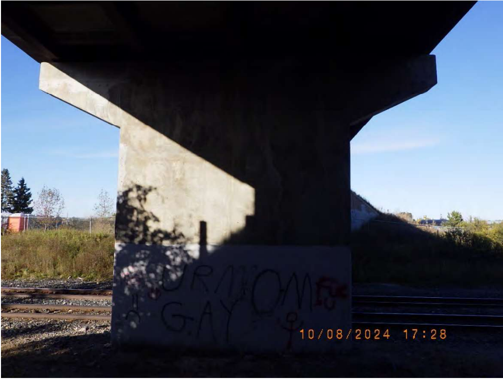
Photo 18: South face of south pier.
