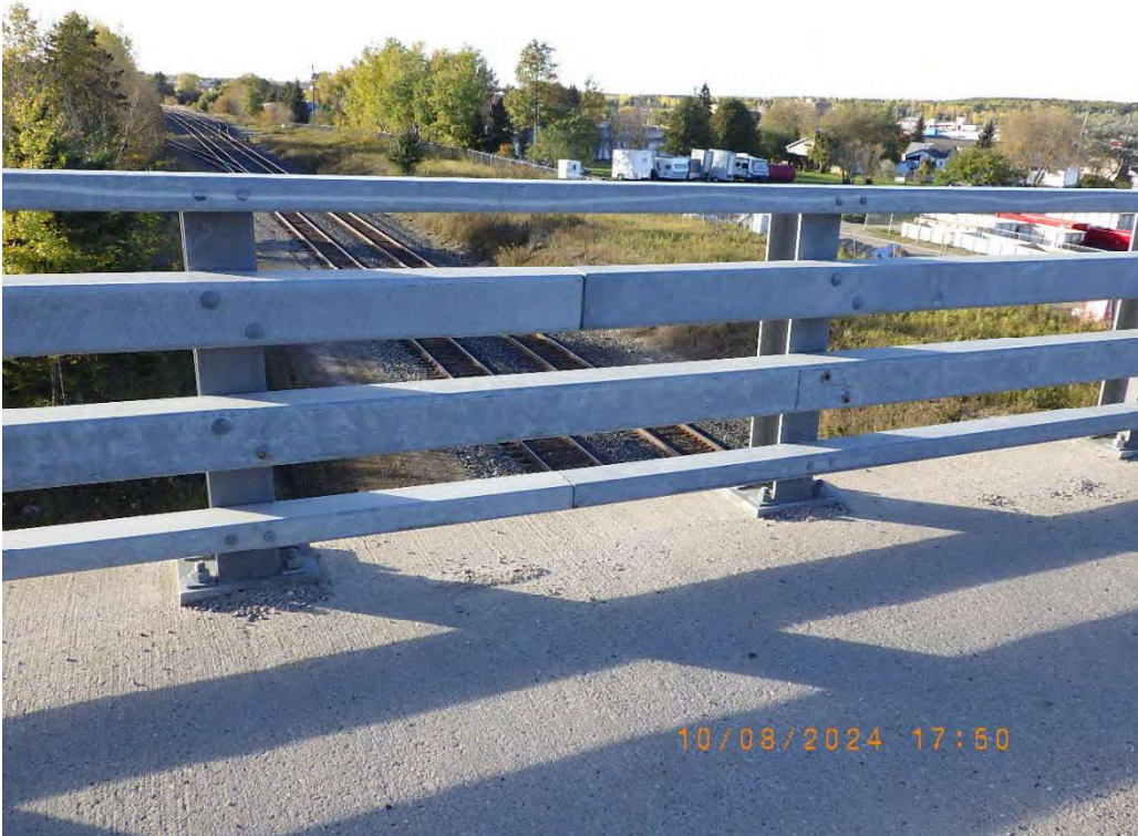
Photo 28: Barrier rail along west side of bridge.
