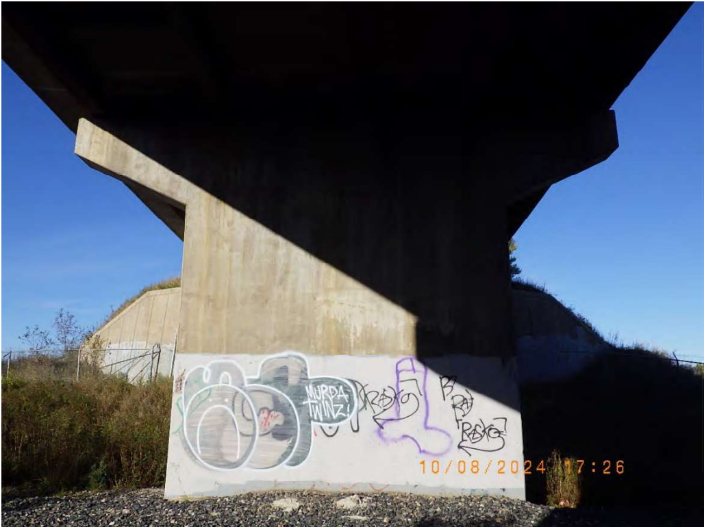
Photo 16: South face of north pier.
