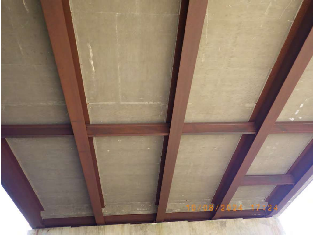
Photo 8: Underside of deck at north span.
