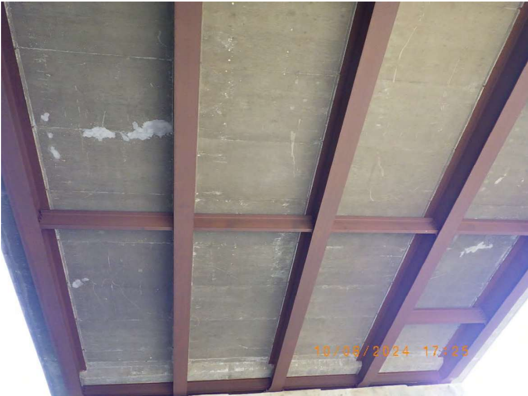
Photo 7: Underside of deck at middle span.
