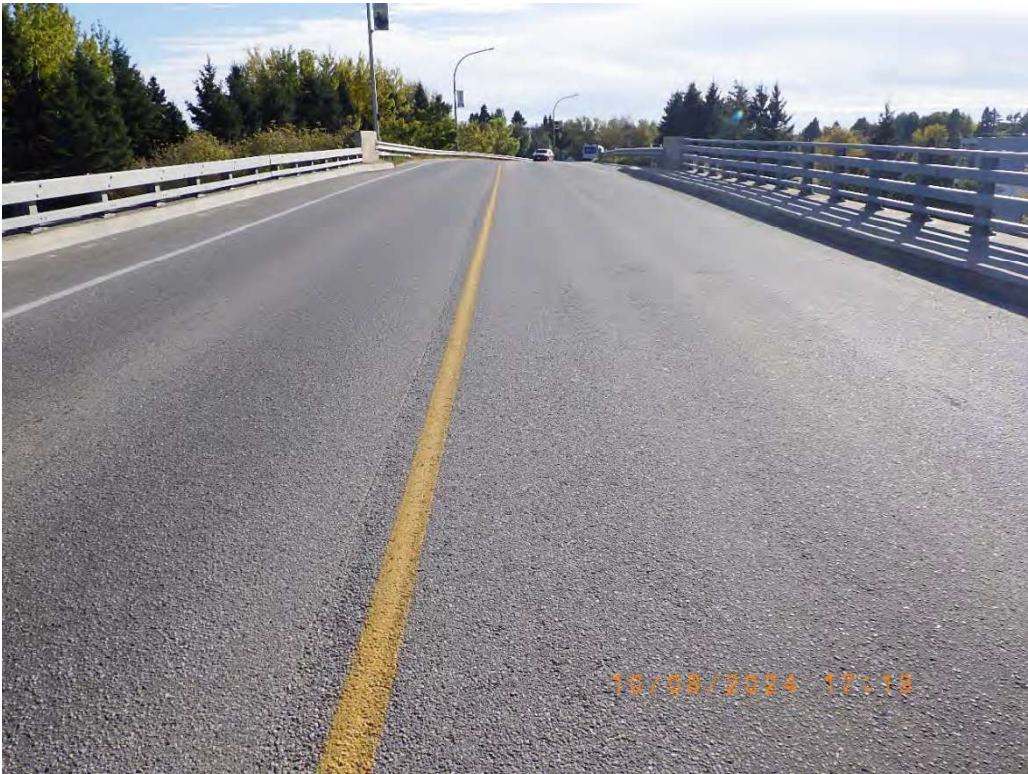
Photo 1: North approach to bridge.
