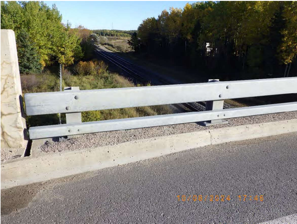
Photo 27: Barrier rail along east side of bridge.
