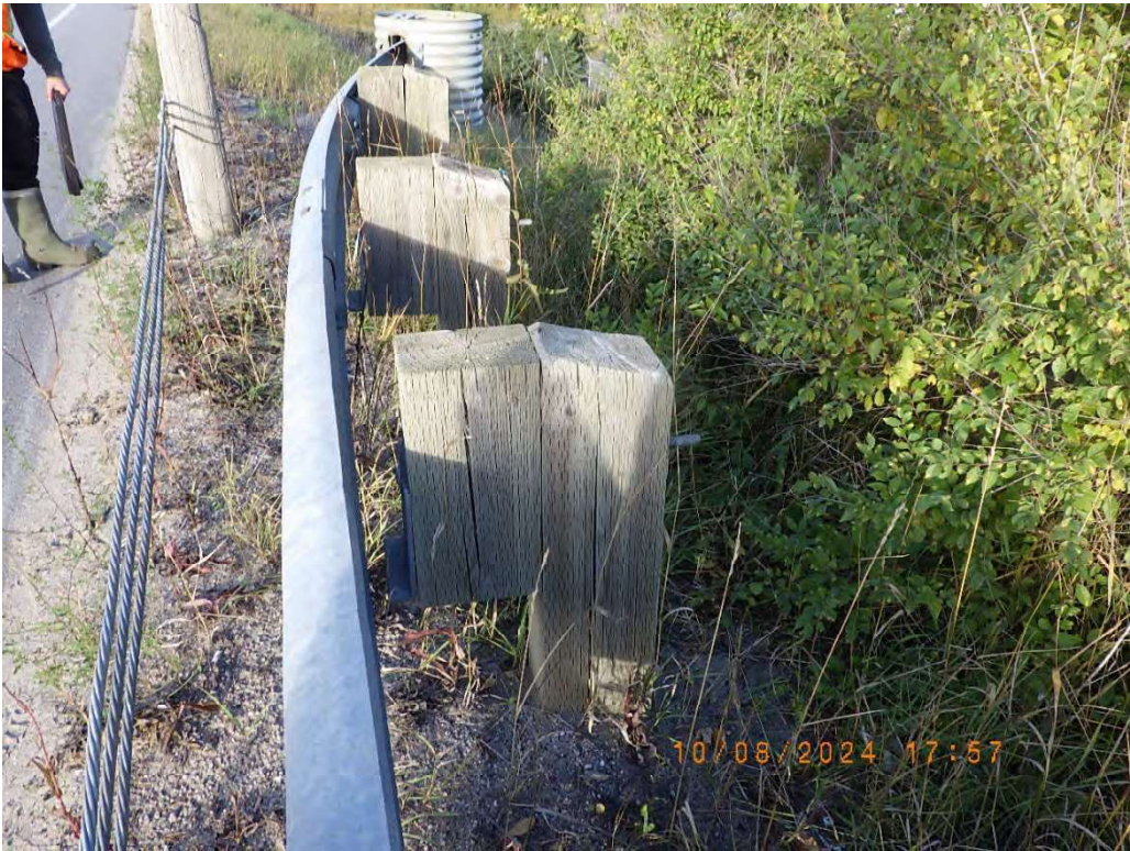
Photo 39: Steel beam guide rail off steel shelves at northeast end treatment.
