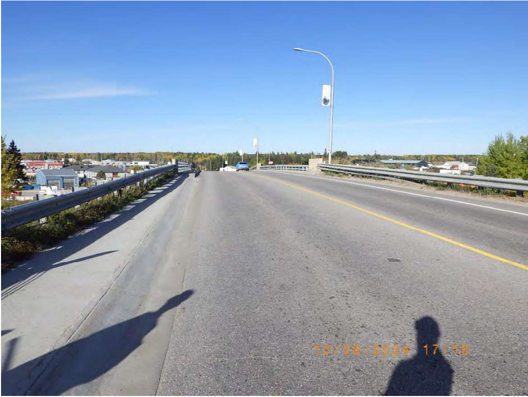
Photo 2: South approach to bridge.
