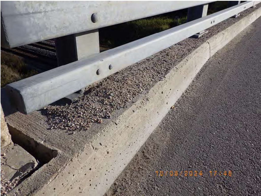
Photo 31: Gravel accumulation on curb and post base plates.
