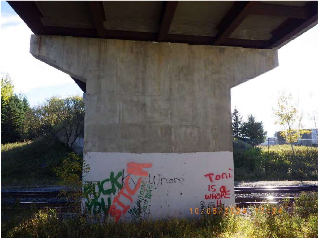
Photo 15: North face of north pier.
