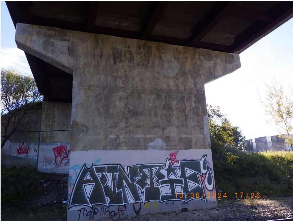
Photo 17: North face of south pier.
