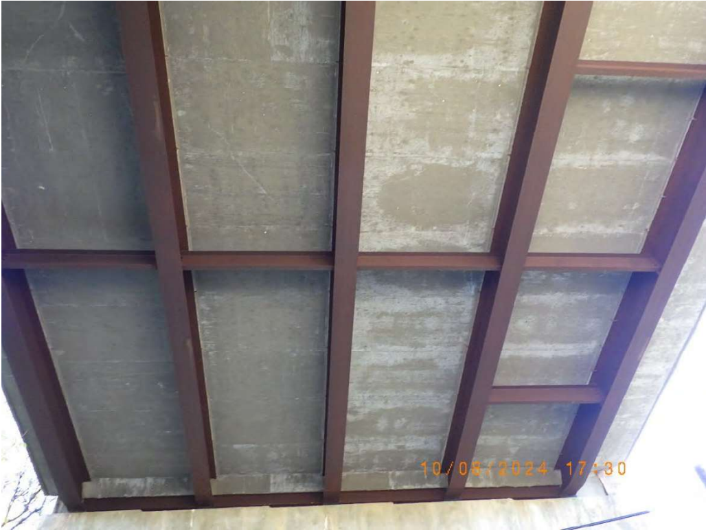
Photo 6: Underside of deck at south span.
