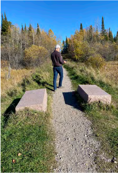
Photo 20: Granite quarry block vehicle deterrents
