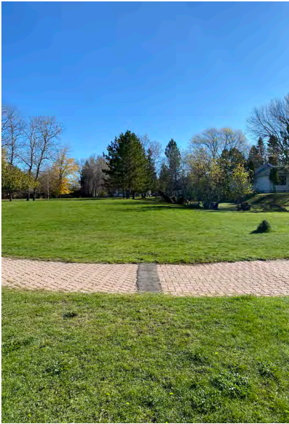
Photo 5: Asphalt patch on trail
