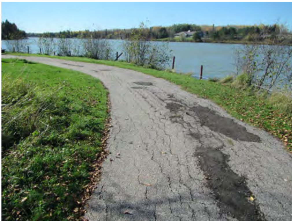
Photo 6: Patched Asphalt Trail Section just North of Skene Landing
