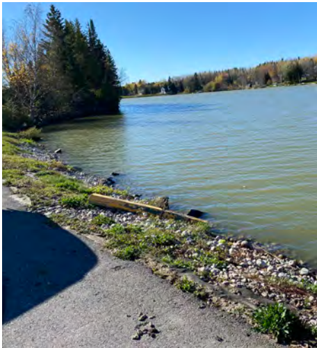
Photo 11: Curb stops pushed into river
