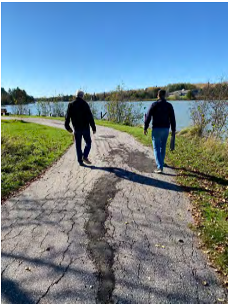
Photo 9: Uneven areas of asphalt trail
