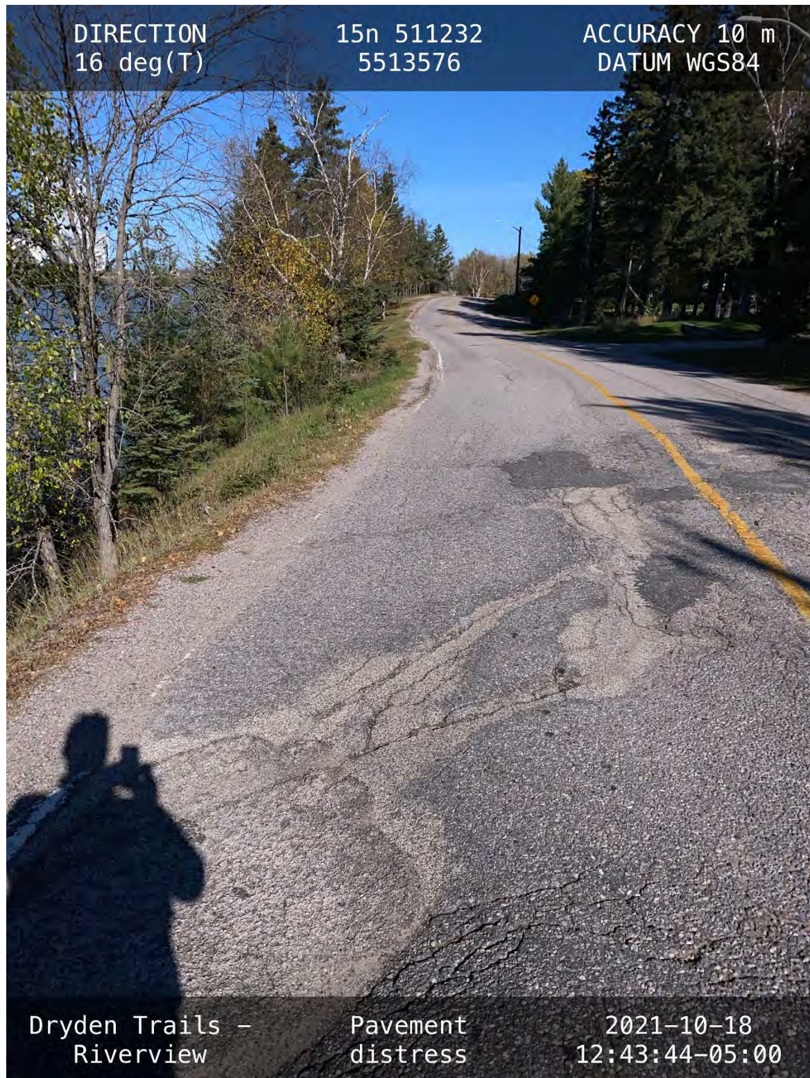
Photo 8 – Pavement distress due to slope creep movements in Section 3 (Riverview Drive)
