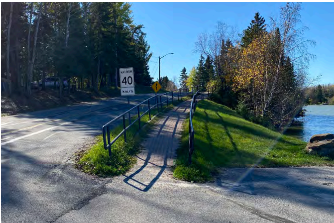
Photo 12: Unit paver ramp up to roadside section of trail
