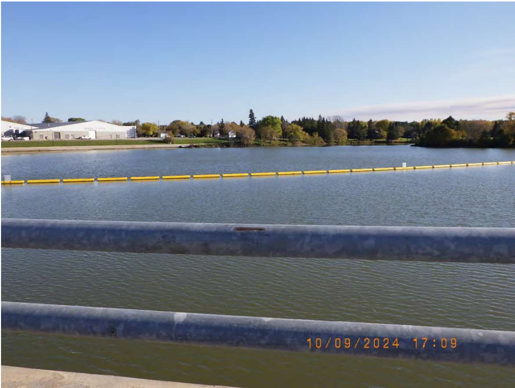
Photo 10: Upstream view from bridge.
