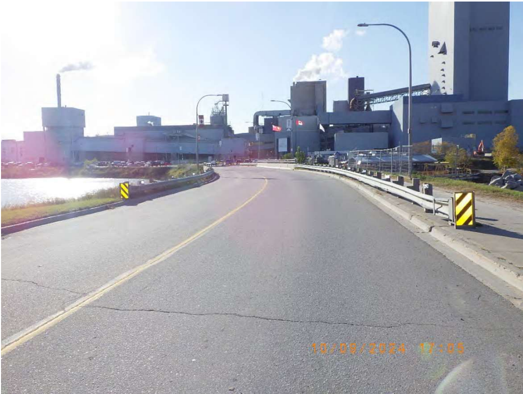
Photo 1: East approach to bridge.
