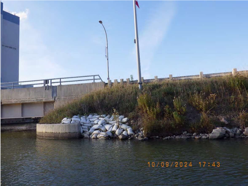
Photo 29: Sandbags at base of southeast embankment.
