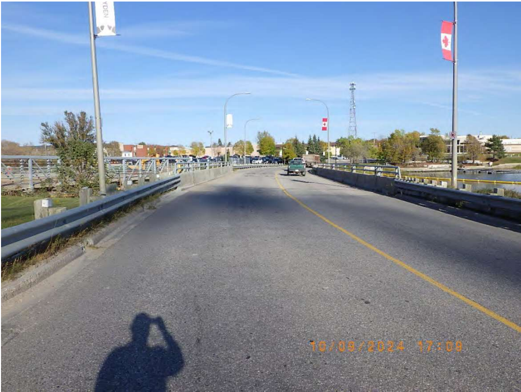
Photo 2: West approach to bridge.
