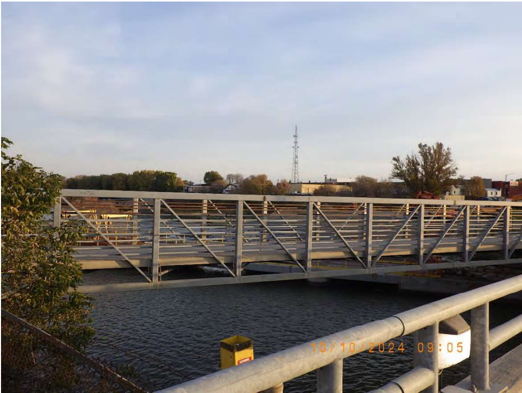
Photo 9: Downstream view from bridge.
