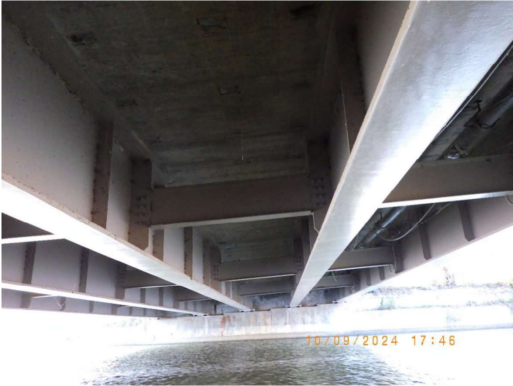
Photo 6: Underside of bridge.
