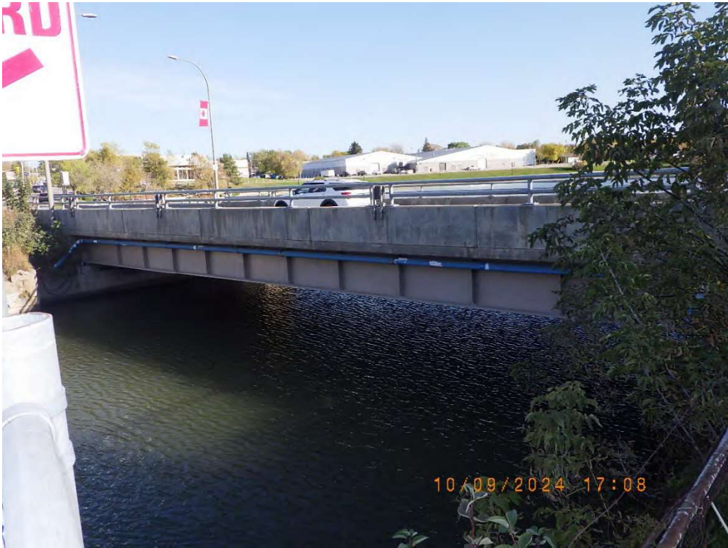
Photo 4: Downstream elevation looking south.
