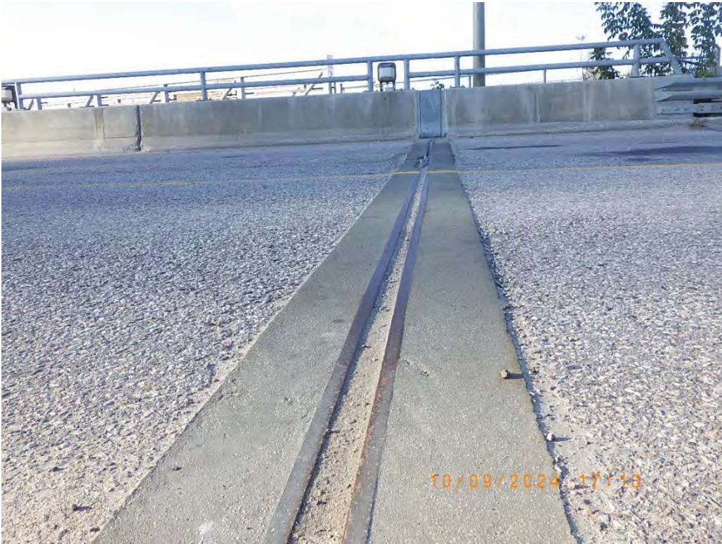
Photo 11: East expansion joint.
