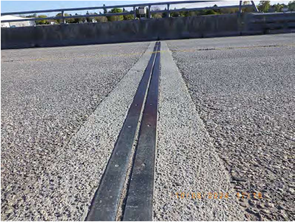
Photo 12: West expansion joint.
